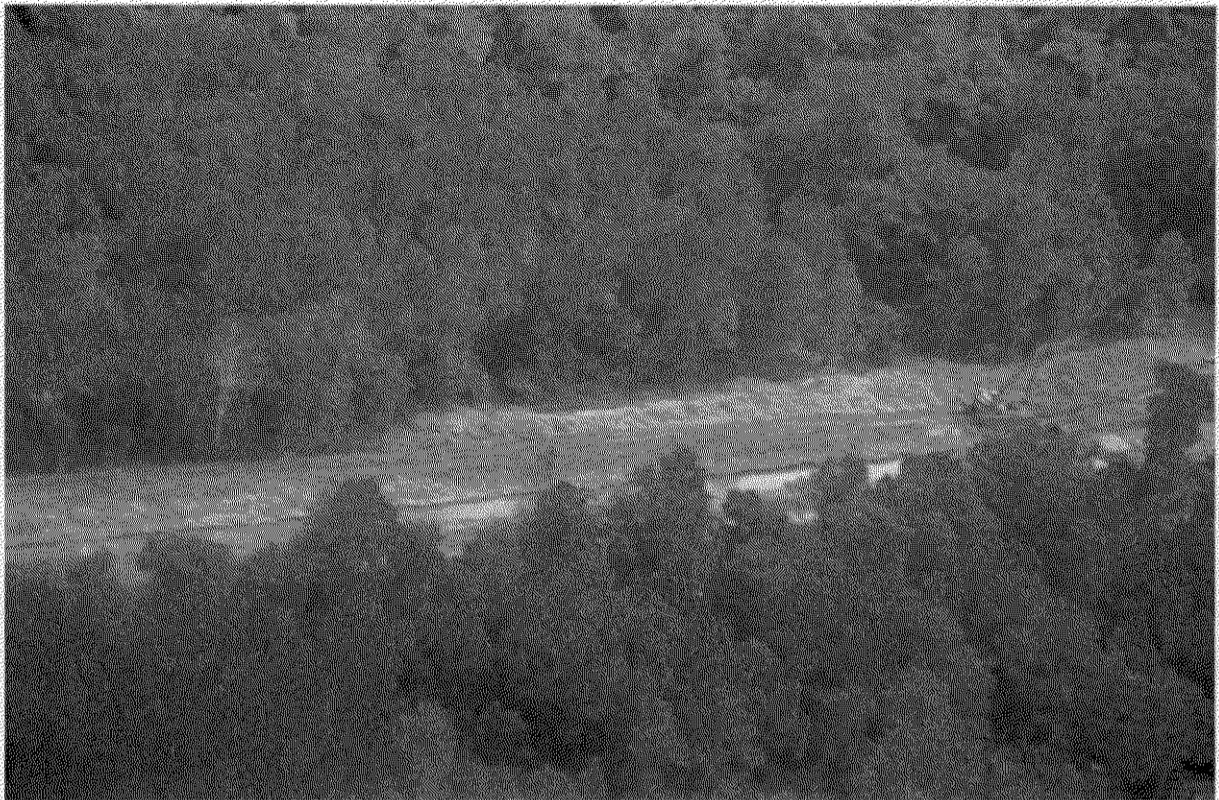
Figure 3. This photo was taken by Dean Wilson during a monitoring flight on July 23, 2018. This photo depicts the pipeline right of way as it crosses the Property. As seen in the photo, there is equipment on the Property and it appears that the trench in which the pipe will be laid is being dug along the pipeline route as it crosses the Property.
