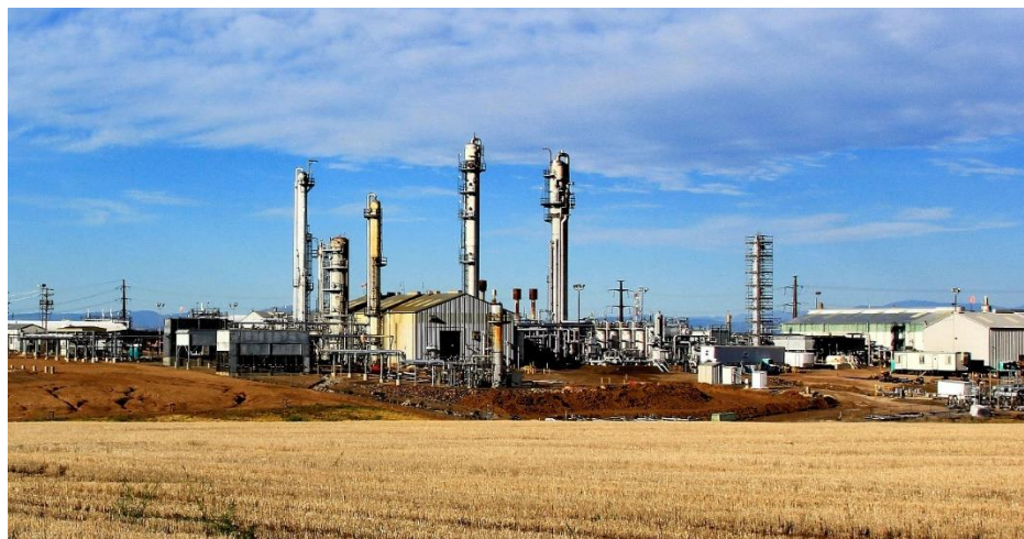
Gas Processing Plant Near Denver, Colorado. Credit: Reid Neureiter/Flickr
